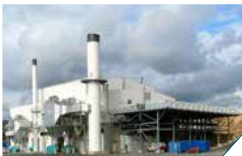
Image detailing the CHP plant and emission control systems
