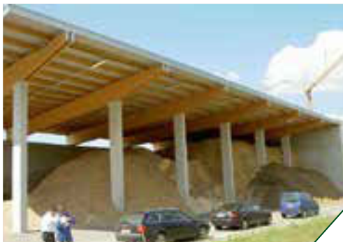
Image detailing the covered fuel yard of the dairy plant
